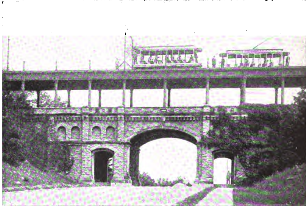
VIADUCT, CINCINNATI, OHIO. (By permission, from the "Scientific American.")
