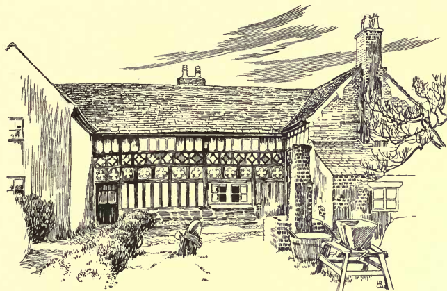
HARLETON HALL: NORTH SIDE OF HALL
