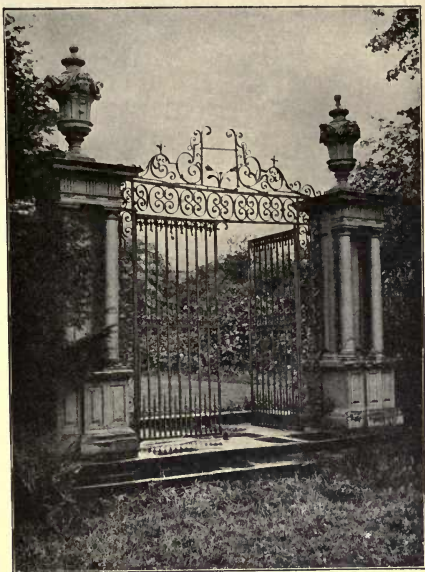
WROUGHT-IRON GATES, CRONTON HALL
