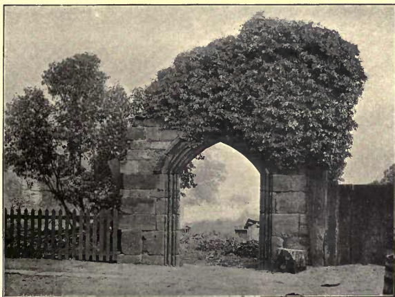
THE OLD HUTT, HALEWOOD : ENTRANCE DOORWAY
