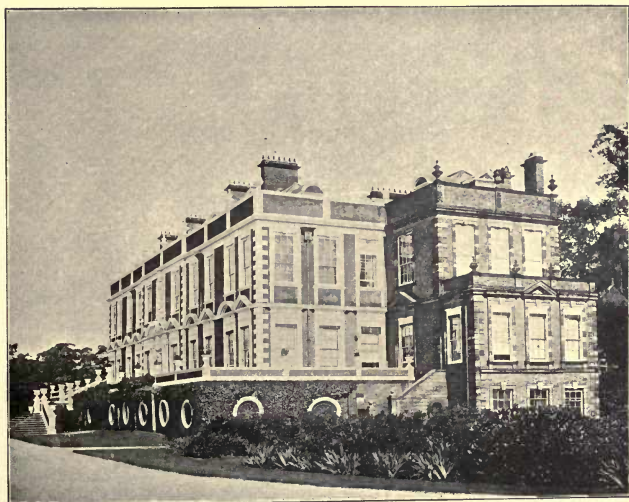
CROXTETH HALL : SOUTH-WEST VIEW
