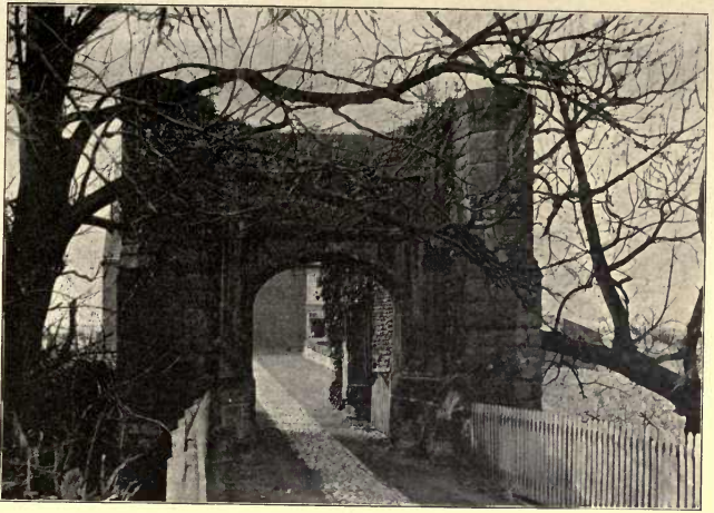
BRADLEY HALL : OUTER FACE OF GATEWAY
