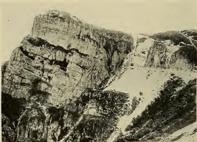
FIG. 123—New Italian military road zigzagging up a steep precipice on the slope of Monte Baldo. Several tunnels may be noted within the space of a few hundred yards.
