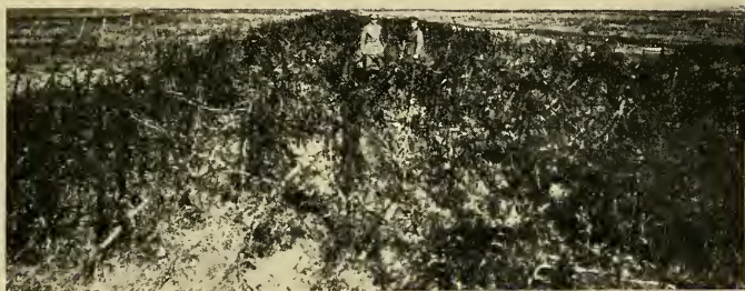
FIG. 47—The main wire defenses of the Hindenburg Line on the chalk plain of the Somme battlefield, southeast of Arras. It was the skillful siting of the defenses on the topography of the plain, more than the formidable entanglements themselves, which gave the famous line its great strength.
