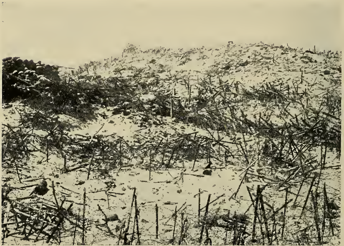
FIG. 20—Barbed wire defenses to prevent an enemy advance along the dry highway formed by the strip of dunes along the coast. Because of the water-soaked character of the maritime plain, the dunes have always been a favorite route for advancing armies. (Belgian official photograph.)
