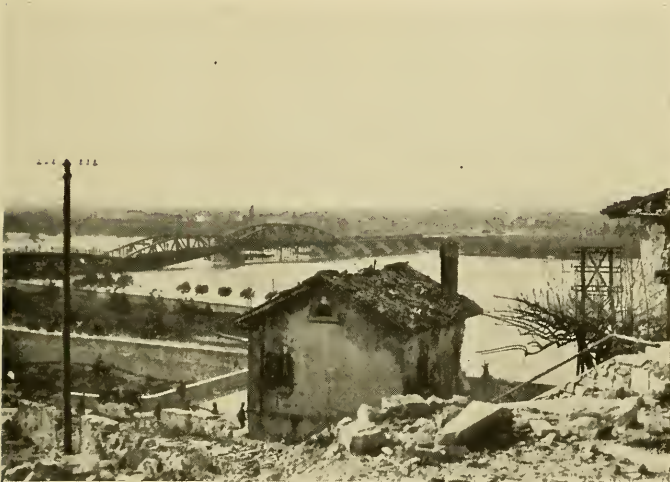
FIG. 150—The Isonzo River at the base of the Carso plateau near Gradisca. The bridge crossing the river has been partially destroyed to prevent easy passage of the barrier. (Italian official photograph.)
