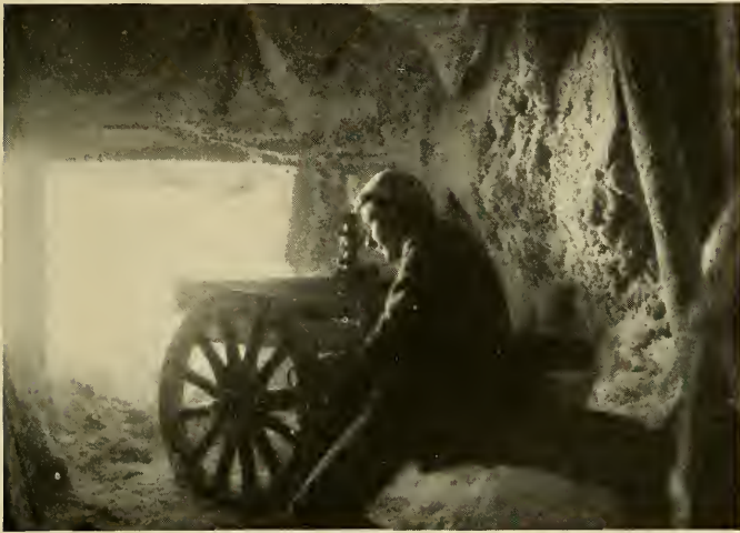
FIG. 139—Gun position at exit of a tunnel excavated in the solid rock of an Alpine mountain. The sides of certain mountains in the Trentino facing the direction of enemy attack were pierced by great numbers of such openings, which transformed the natural obstacles into almost impregnable fortresses. (Italian official photograph.)
