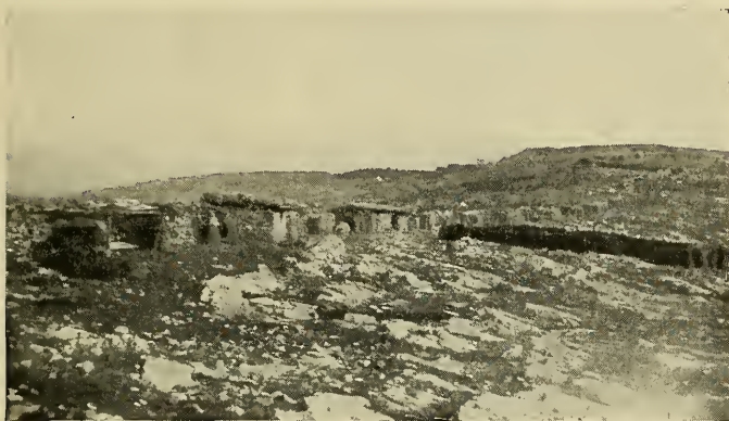
FIG. 147—Defensive position on western margin of the Carso north of Monfalcone. The barren aspect of the limestone country is apparent, and stone breastworks and shelters replace trenches and underground dugouts. (Italian official photograph.)
