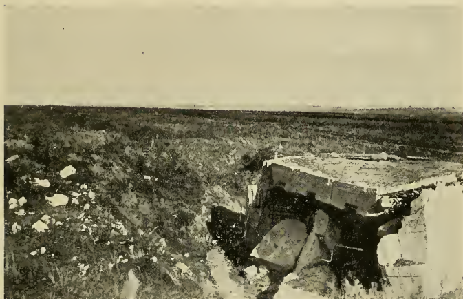
FIG. 54—Partially destroyed concrete machine-gun shelter in a trench of the Hindenburg Line southeast of Arras. From this shelter a deadly grazing fire swept the exposed surface of the barren Somme plain.
