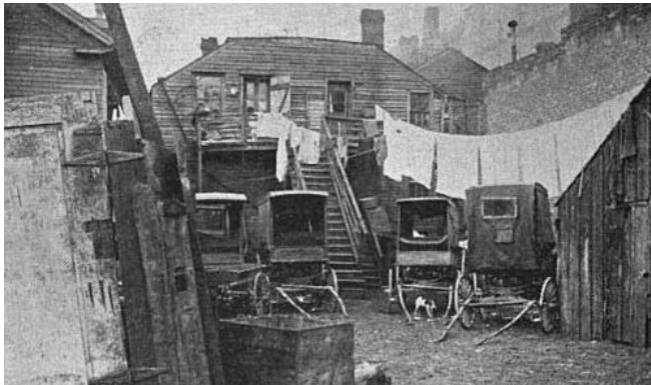
Photo 1.2: Jefferson Street. The shed barn at right contains three horses. The barn next in view contains six horses and two goats. The house in the center of the picture is full of Italian families and presents no redeeming feature. On the left are other tenements full of families. (1911)
