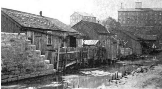
Photo 1.1: Syracuse, NY—Shanties Back to an Open Sewer. (1901)
