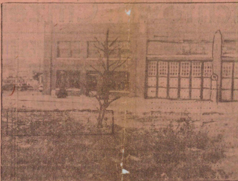
The vacant lot and tree where Matthew Williams was burned by fiends. In the background is the garage where they stole 45 gallons of gas to pour on the dead man's body. This is where the sheriff told the mob he thought they had done enough.
